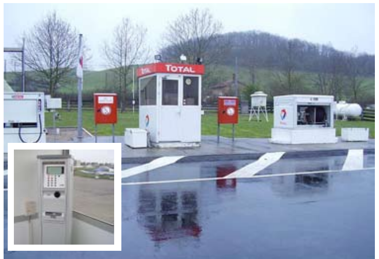
Typical airfield fuelling station in France with the Autofuel Terminal HECFLEET (small picture)..
